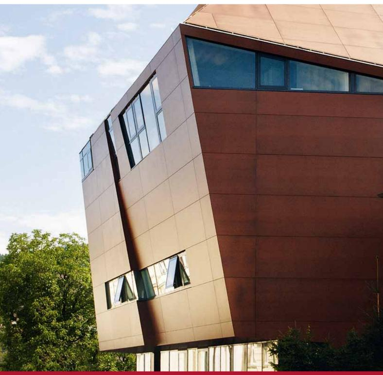
Joint profiles (corrugated profile) vertical and horizontal
